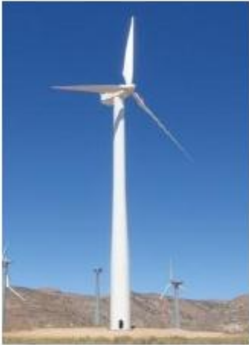
Figure 7 - PS-600 turbine
