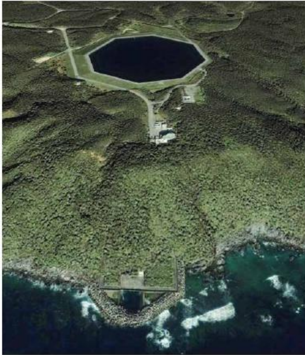
Pumped hydro storage using seawater in Okinawa
